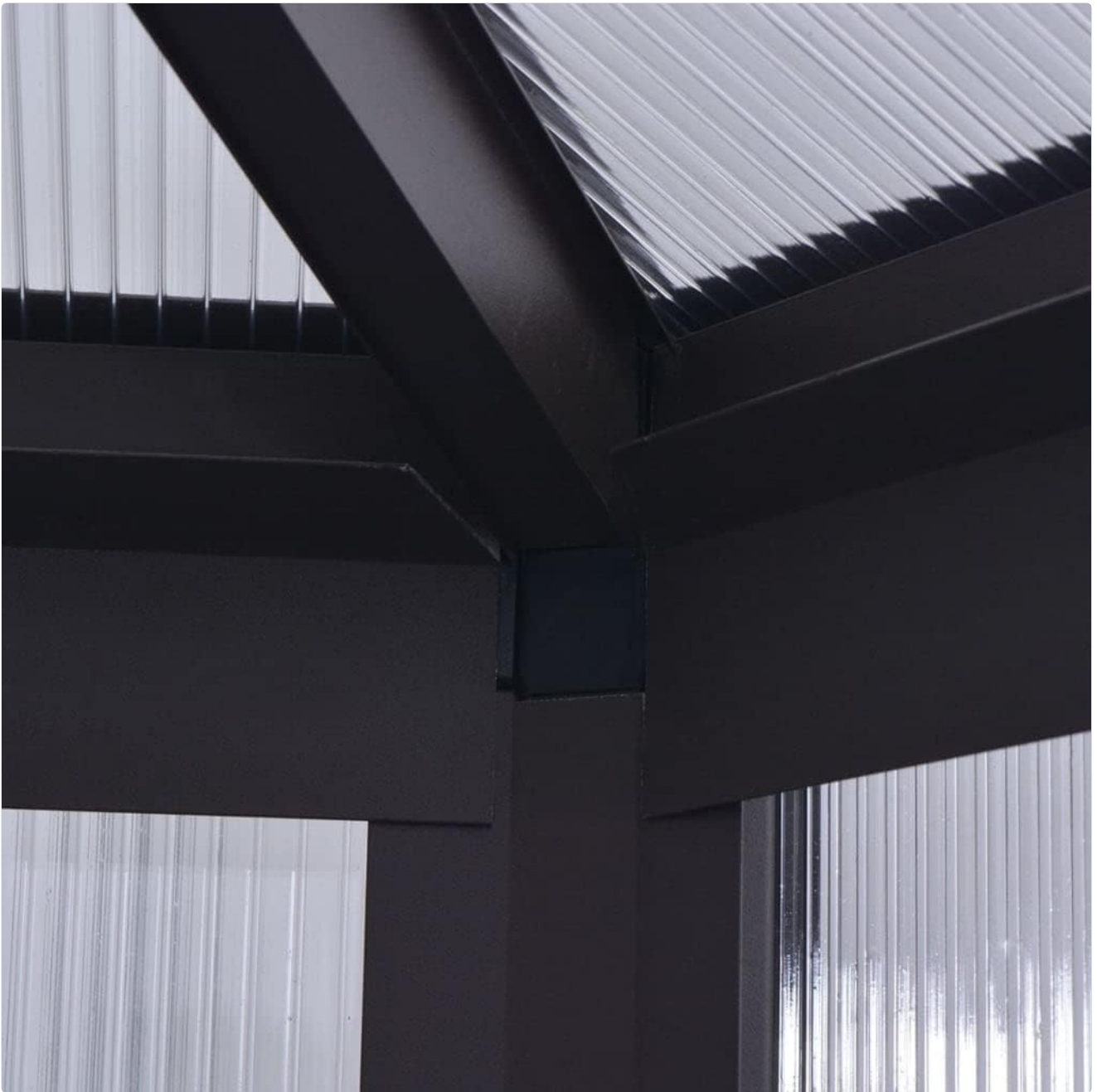
Figure 4.3.1: Example of an upper frame corner joint during assembly.
