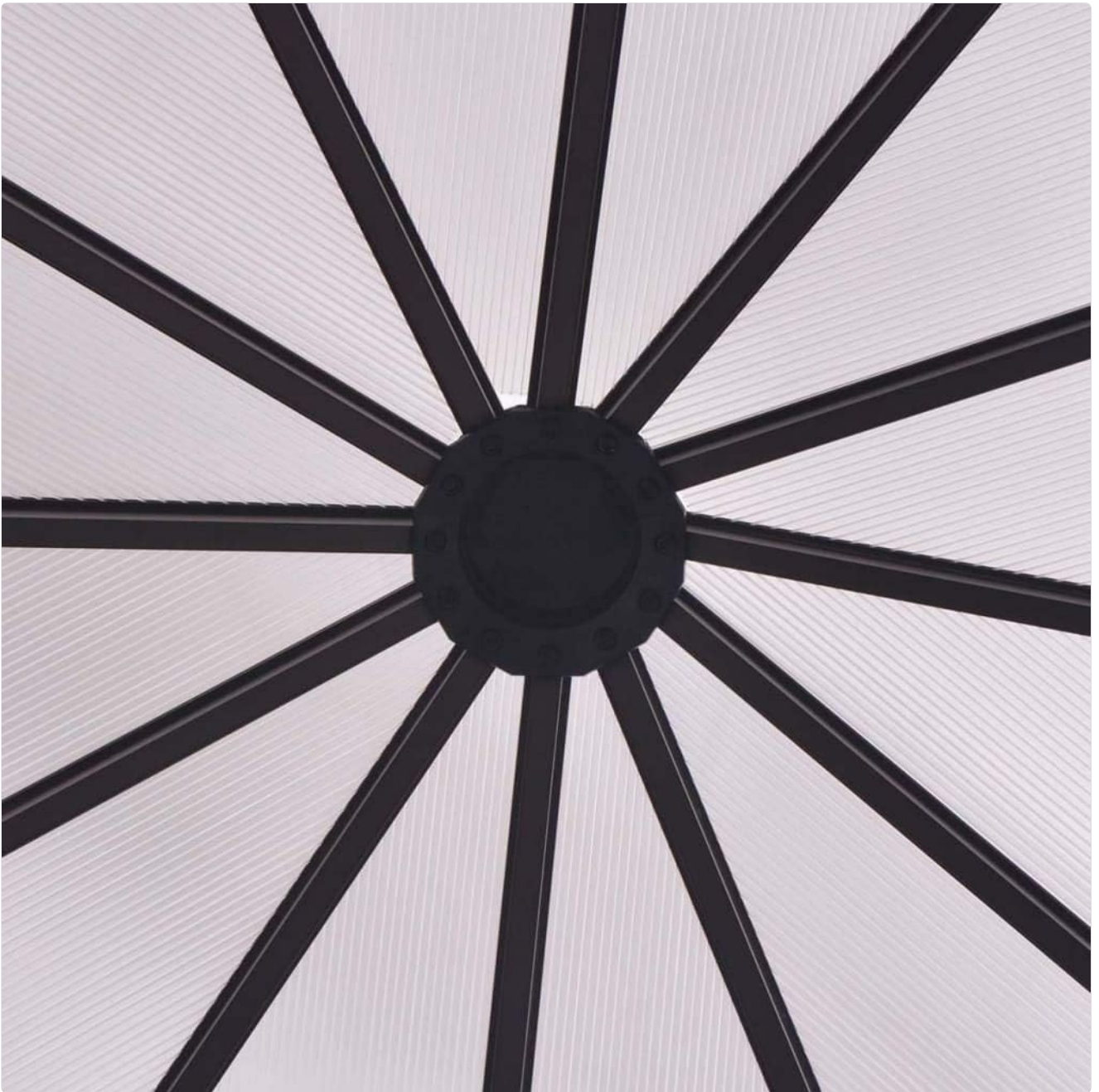
Figure 4.5.1: Interior view of the completed roof structure.
