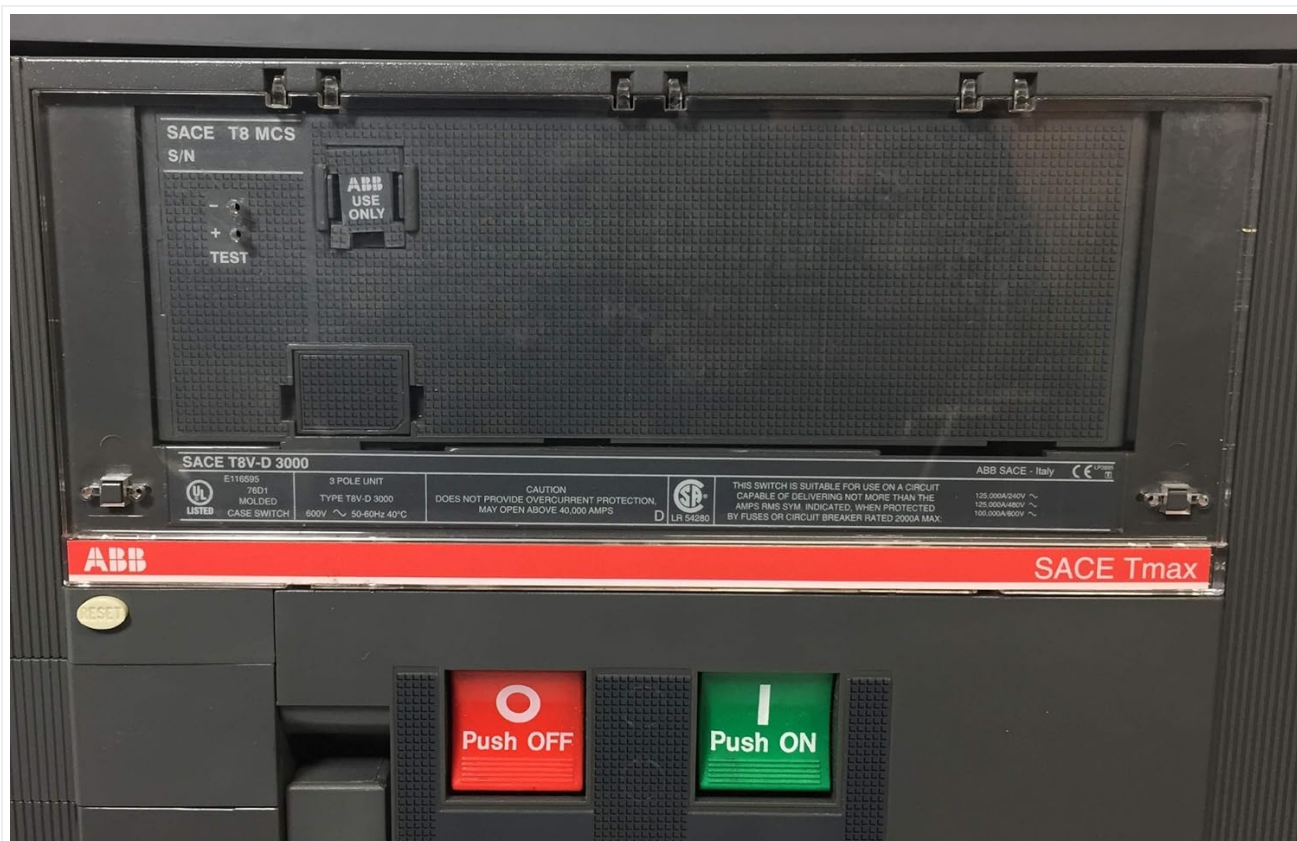
Figure 3.2: Close-up view of the control panel, highlighting the 'Push OFF' and 'Push ON' buttons, and detailed product labels including model number and ratings.
