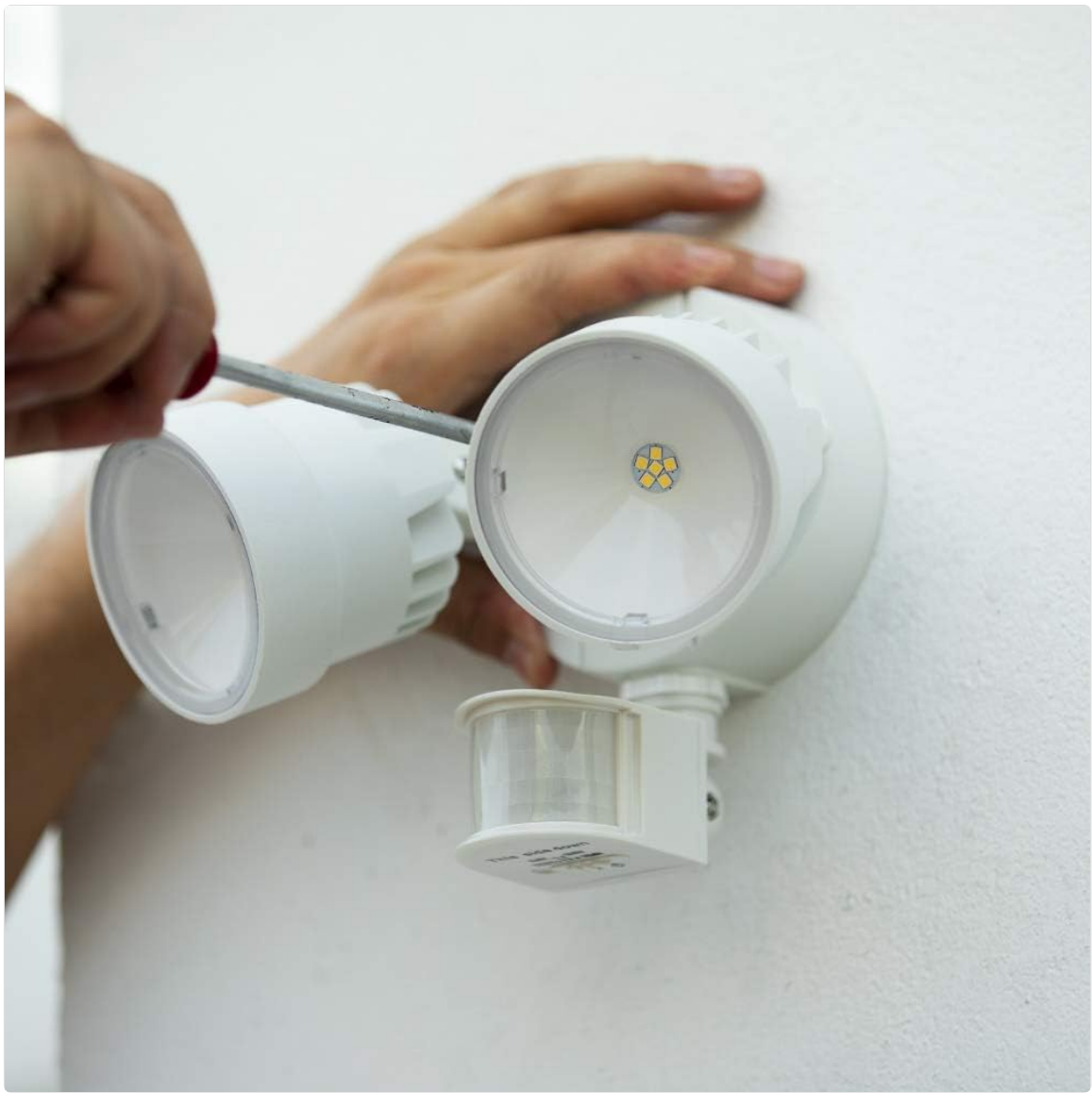
Image 4.1: A person using a screwdriver to secure the floodlight during installation, demonstrating the final mounting step.
