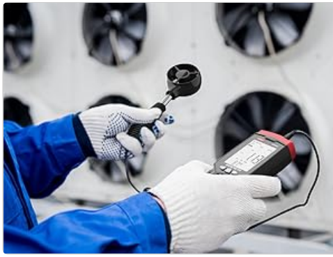
Figure 3: Measuring wind speed and air flow from an HVAC vent.
