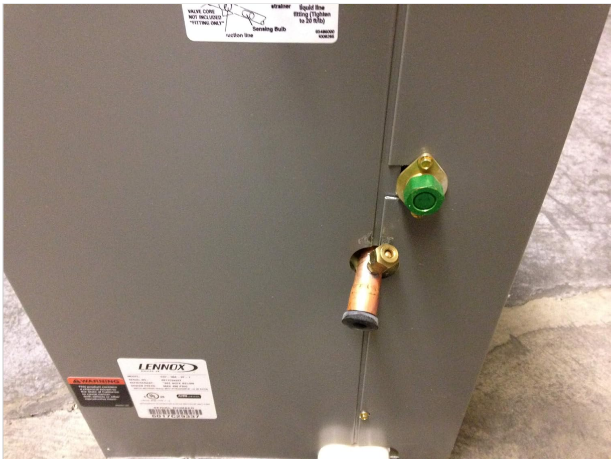
Image: Close-up view of the refrigerant line connections and service ports on the side of the Lennox A-Coil.
