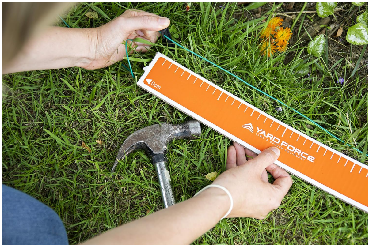
Image: A person uses an orange ruler to measure the precise distance of the boundary wire from the edge of a garden bed, ensuring correct installation.
