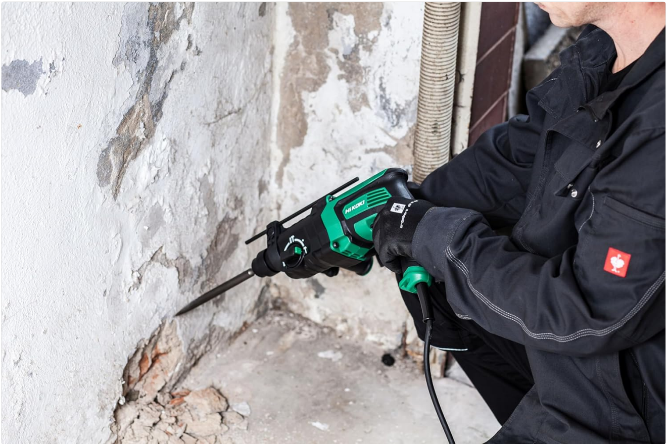
Image 4: Chiselling operation
