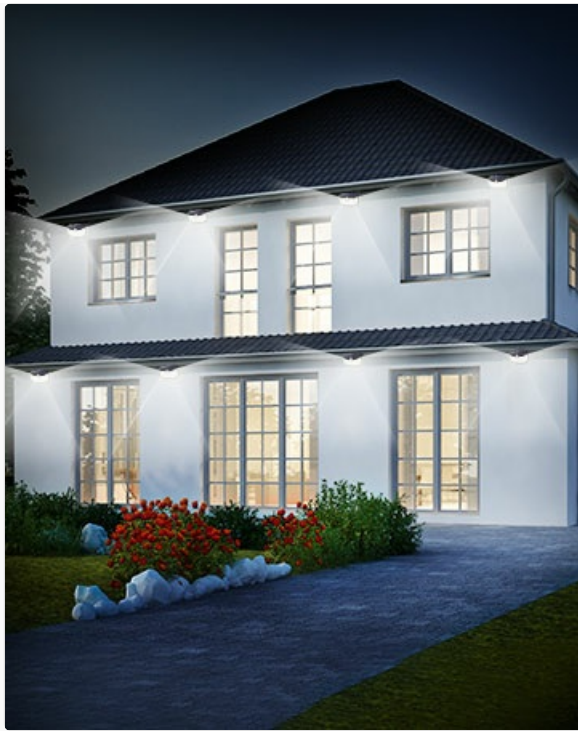
Figure 4: Example Installation on a House Exterior
