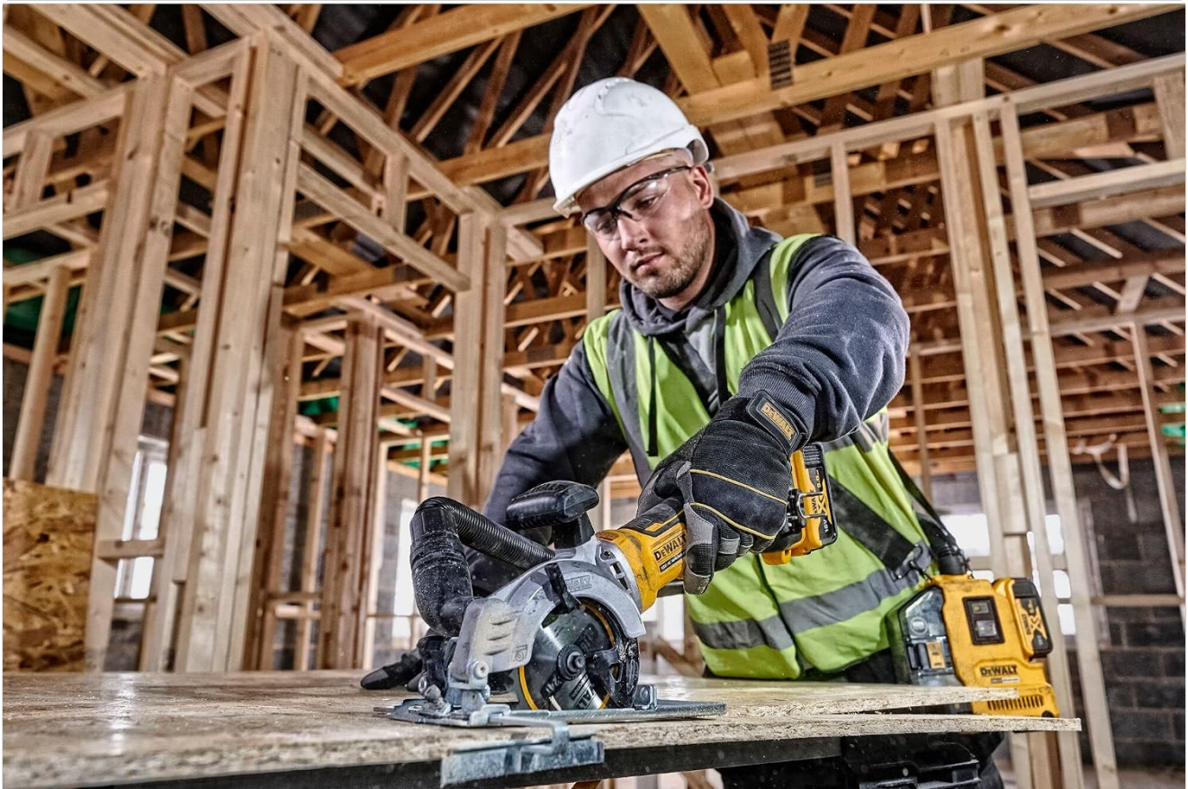
Figure 3: Worker demonstrating proper handling and cutting technique with the circular saw.
