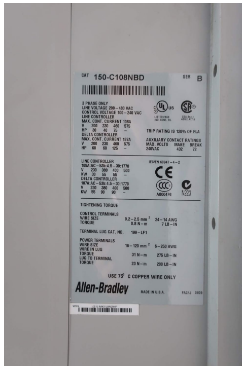
Figure 3.2.6: Detailed view of the product label, showing CAT 150-C108NBD, UL, CSA, CE markings, and detailed electrical ratings for line and delta controller configurations. Also visible is a barcode with the number 21MK1UW2HP and the model number 150-C108NBD B .
