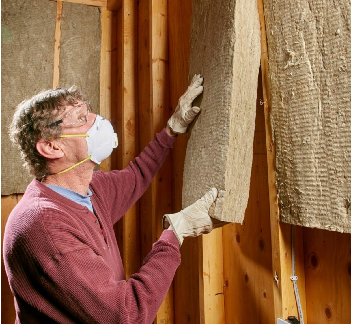
Figure 3: Proper PPE (mask and gloves) during insulation installation.
