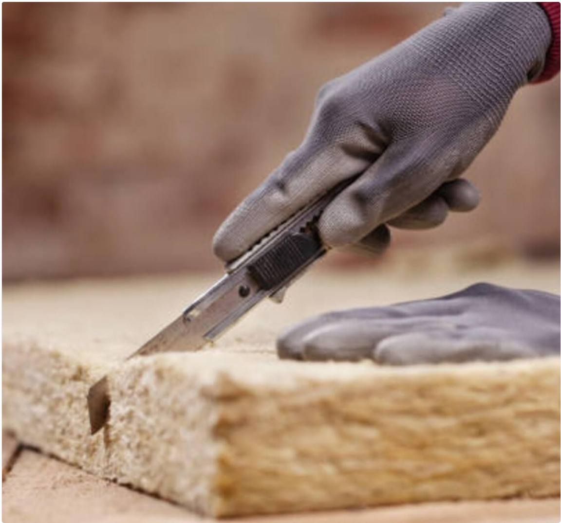
Figure 4: Cutting ProRox SL940 board with a serrated knife.
