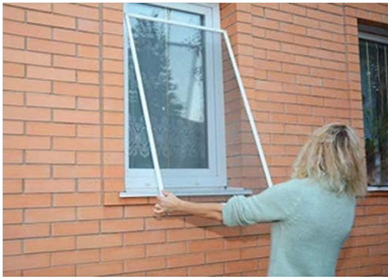
Figure 3: An individual demonstrating the process of installing a pre-framed window screen into a window opening. The screen is lightweight and designed for easy placement.
