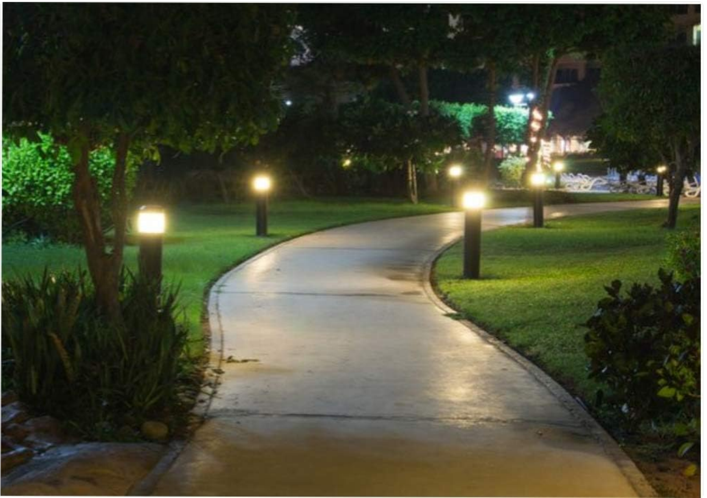
Image: A curved outdoor pathway at night, lit by multiple bollard-style landscape lights, highlighting the consistent light distribution of the bulbs.
