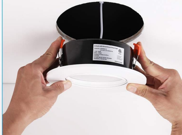
Figure 5.1: Visual guide for the installation process, from cutting the hole to securing the light in the ceiling.
