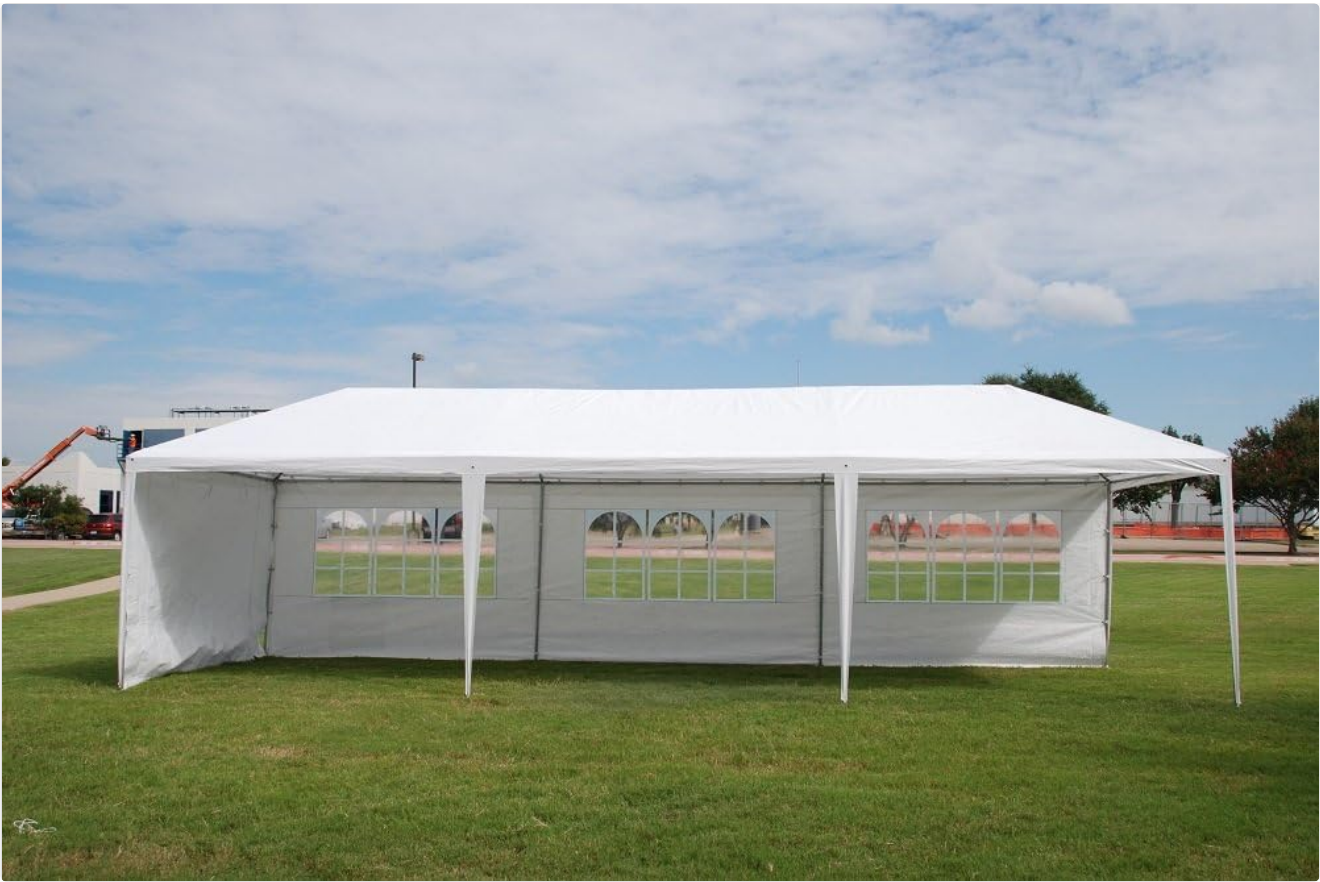
Image 4.2: Tent with roof cover installed, prior to sidewall attachment.
