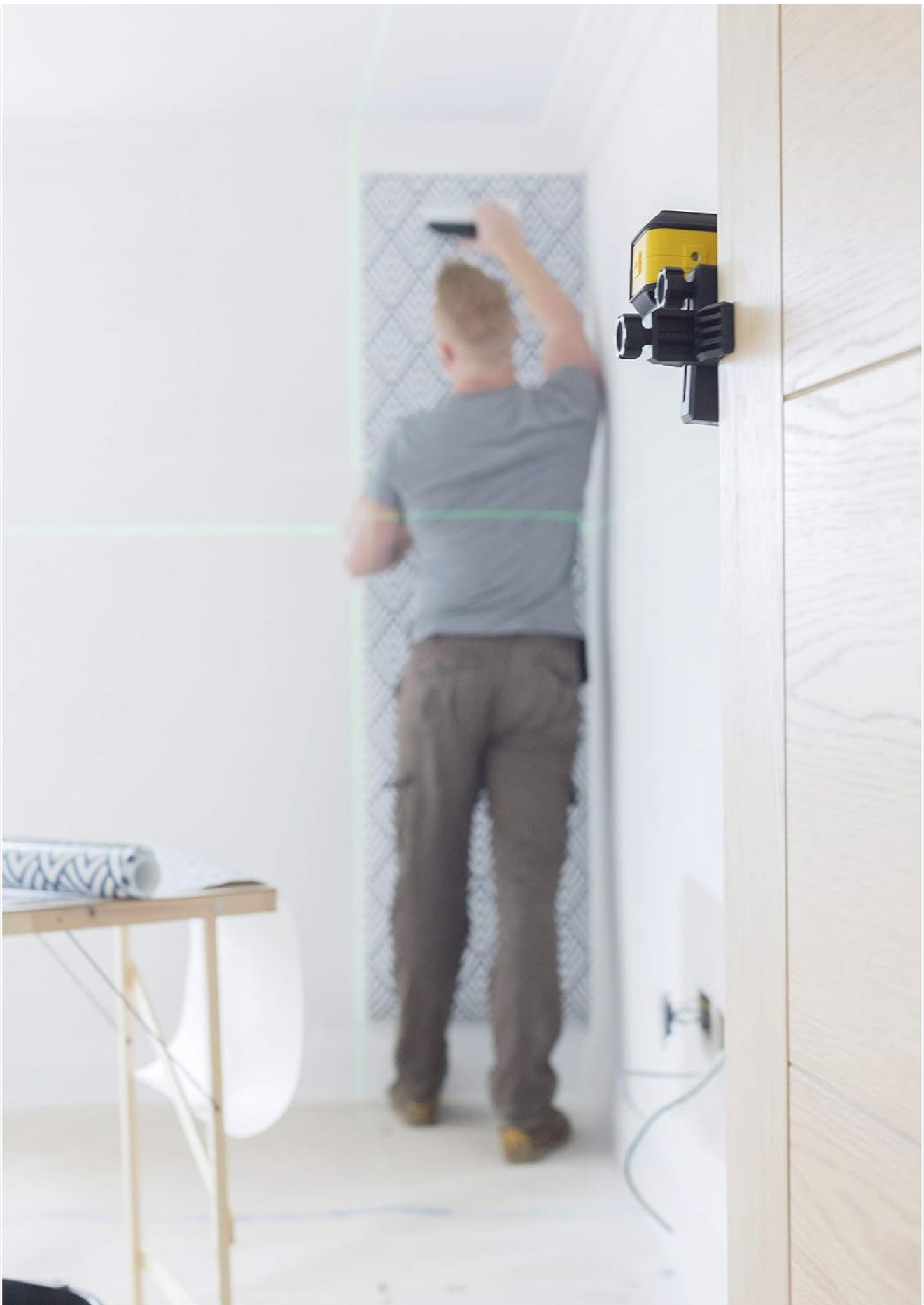
Figure 3: An individual is shown utilizing the Stanley Cubix laser level to project precise horizontal and vertical green laser lines onto a wall, aiding in the accurate alignment of wallpaper during installation.
