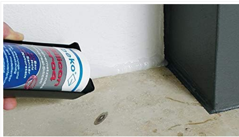
Image 4.3: Sealing a joint between a floor and a wall, showcasing the product's flexibility for various surfaces.
