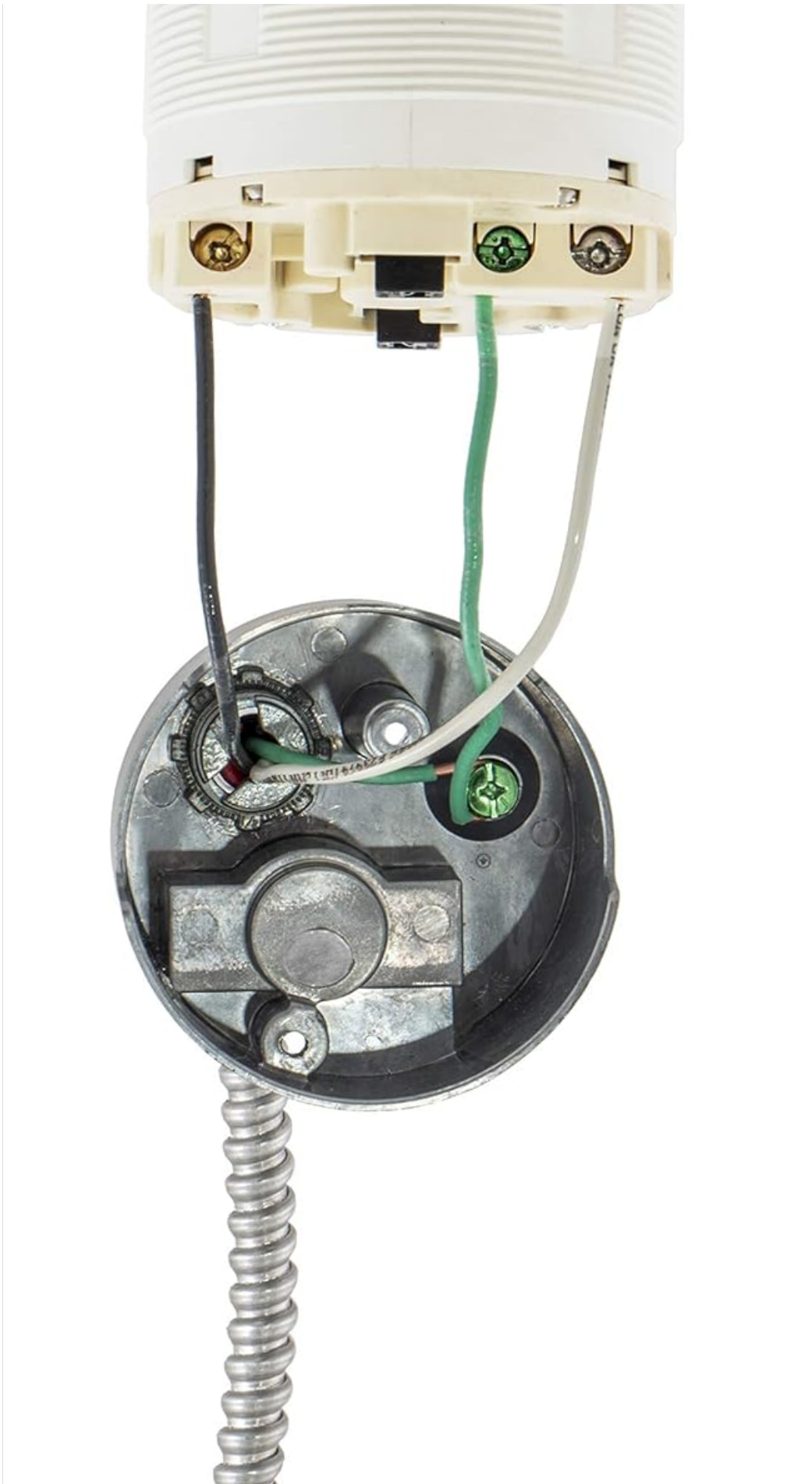
Figure 5: Wiring connections with flexible conduit.
