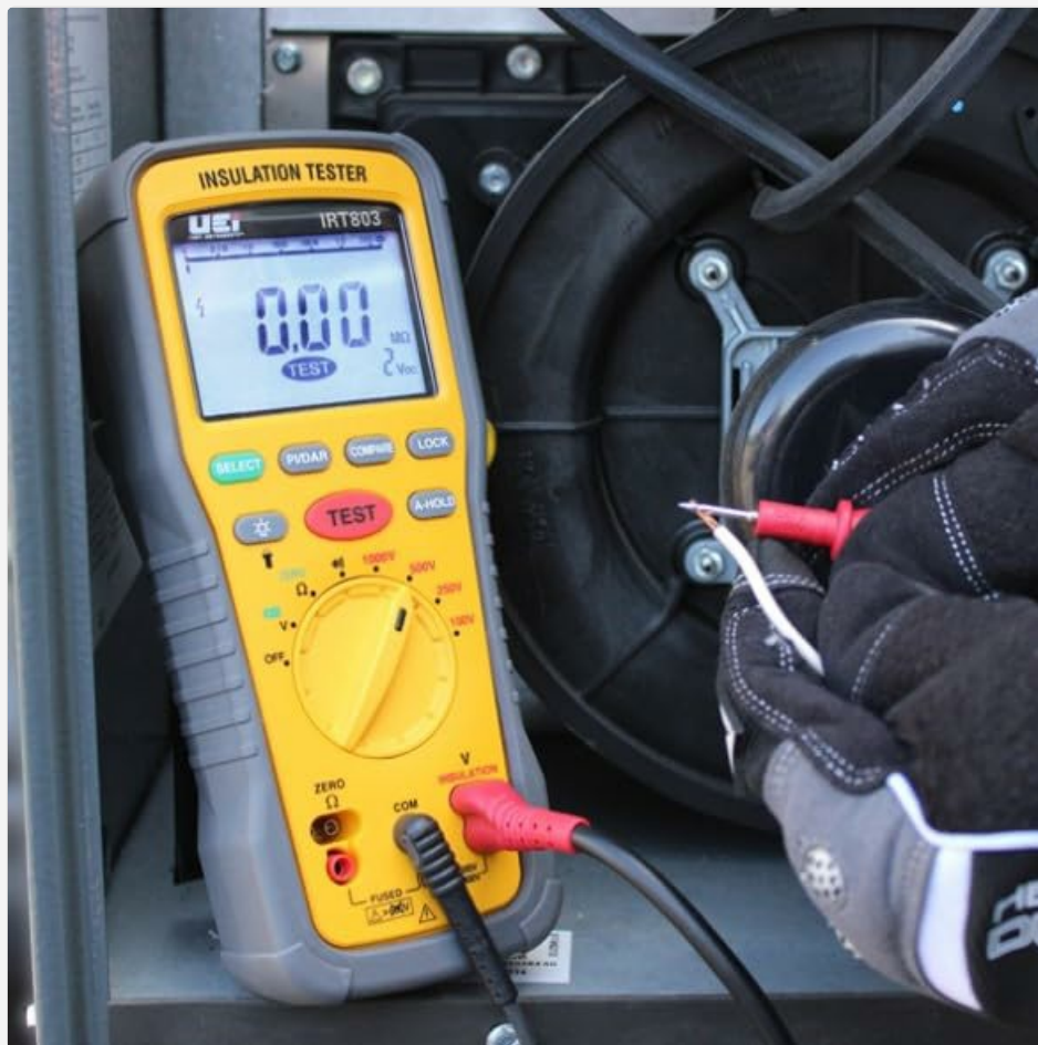
Image 6.1: The IRT803 being used to measure insulation resistance on electrical wiring.
