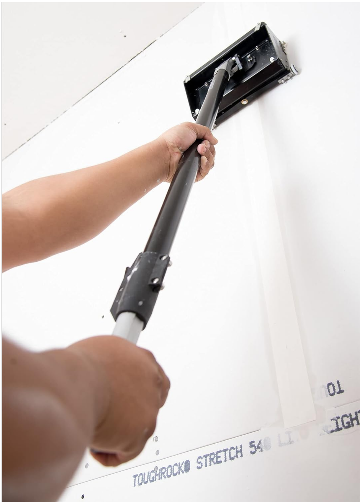
Image 2: A user demonstrating the application of joint compound with the DEWALT Flat Box Extension Handle.
