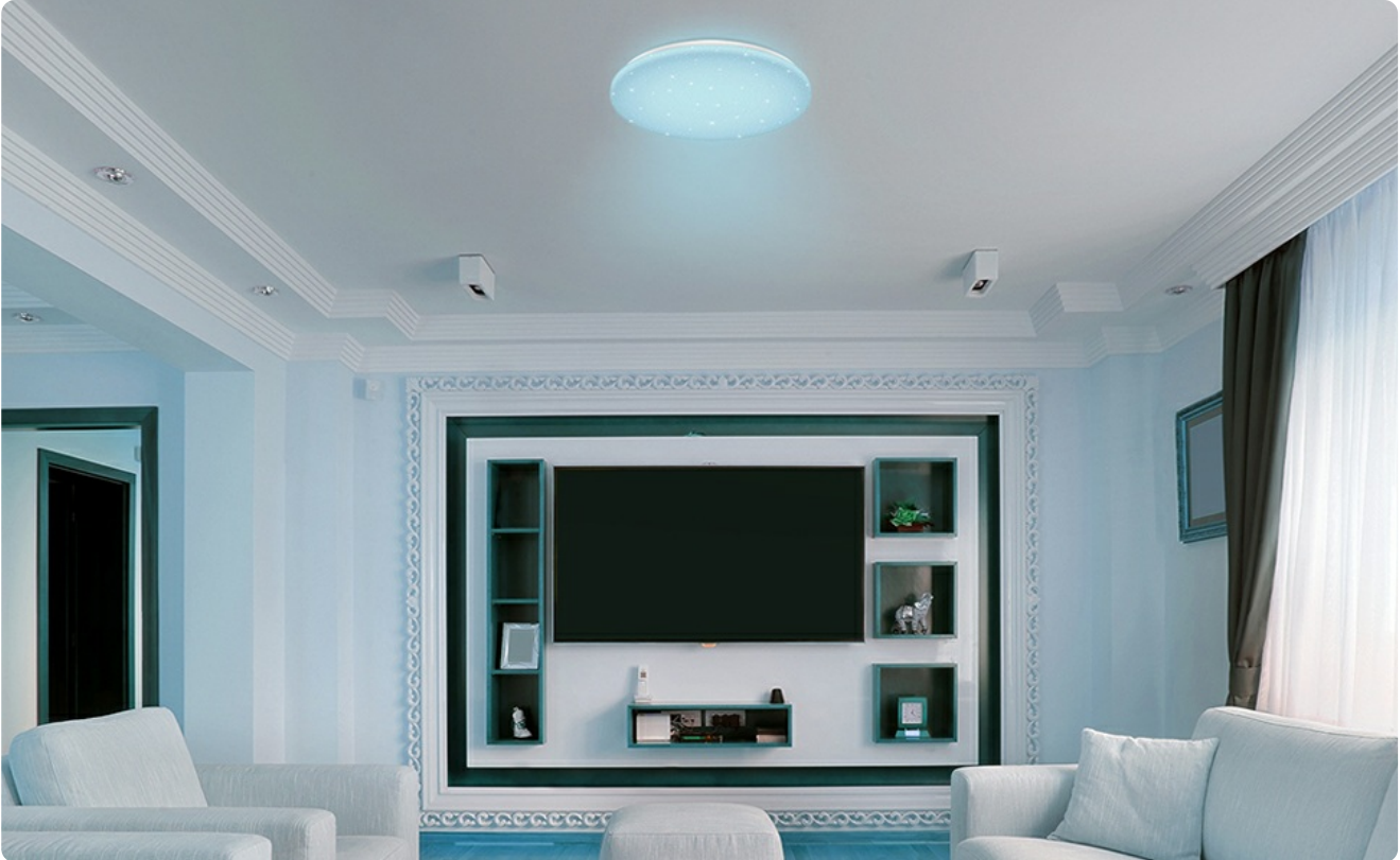
Image: The Horevo ceiling light installed in a modern living room, demonstrating its aesthetic integration.
