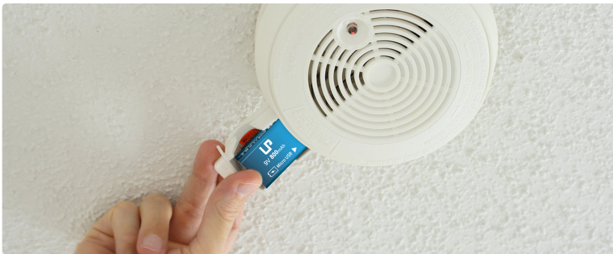
Image 3: A hand demonstrating the insertion of an LP 9V battery into a smoke detector.
