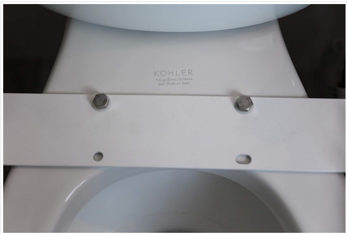
Image 4.2: Top-down view showing the white mounting bracket of the TILT lift secured to the back of a toilet bowl, with two bolts visible.
