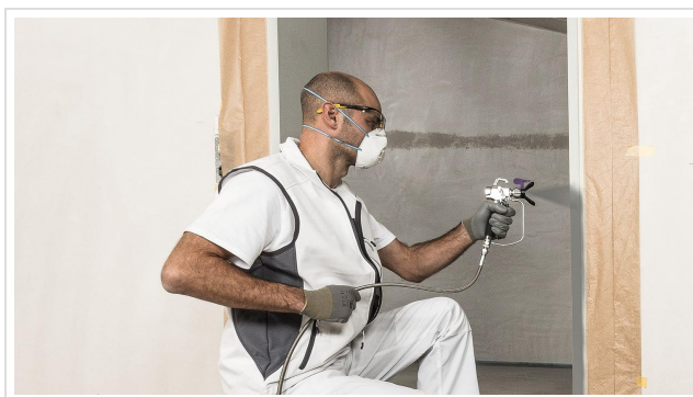
Image: A person wearing protective gear, using an airless sprayer with a Wagner nozzle to paint an interior wall, demonstrating application in a confined space.
