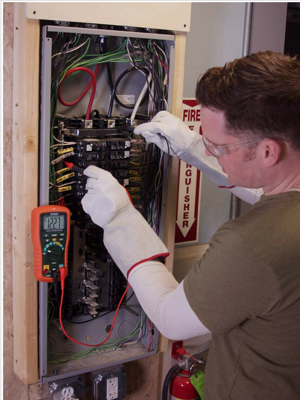
Figure 4: An electrician safely measuring voltage within an electrical panel using the Extech MM750W Multimeter. The meter's display is visible, showing a reading.
