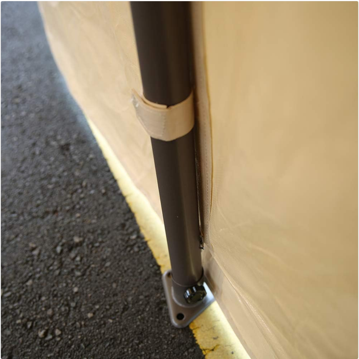
Figure 2: Base plate and pole connection for ground stability.
