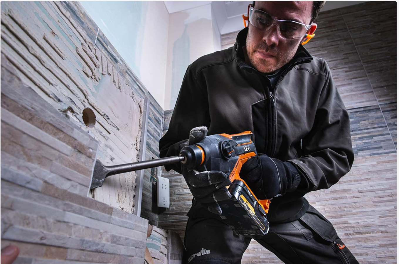
Figure 7: Worker performing chiseling work on a wall, demonstrating the tool's hammer function for material removal.
