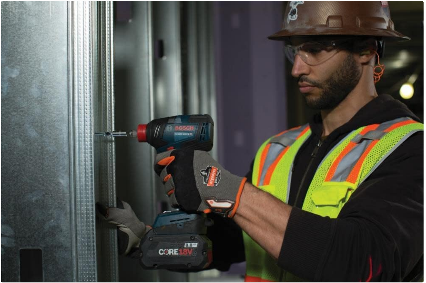
Figure 3: A construction worker utilizing the Bosch GDX18V-1800CN impact driver to secure a fastener into a metal stud, demonstrating its application in professional settings.
