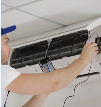
Air conditioning Inspection
