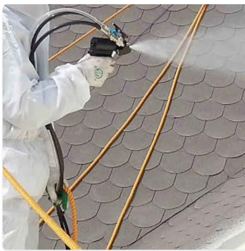
Figure 5: An operator demonstrating the application of foam using the TECHTONGDA P2 spray gun on a roof surface.
