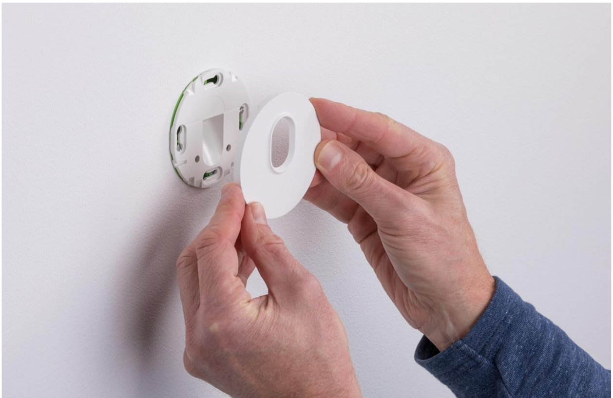
Image 4.3: Hands carefully positioning the white round front cover onto the Paulmann 92924 recessed fixture, completing the installation.
