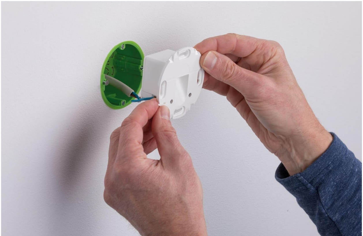
Image 4.2: Hands guiding the Paulmann 92924 fixture into a green electrical box recessed in a white wall, showing the connection process.
