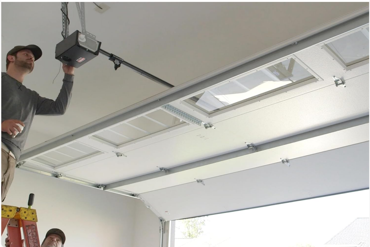
Figure 2: Installation Process. This image shows a person installing the garage door opener unit on the ceiling of a garage, demonstrating the ease of setup.
