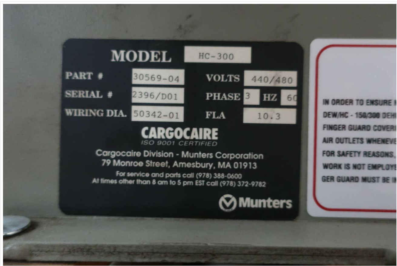
Figure 3: Detailed view of the Munters HC-300 specification label, indicating model number, voltage (440/480V), phase (3), frequency (60 Hz), and full load amperage (10.3 FLA).
