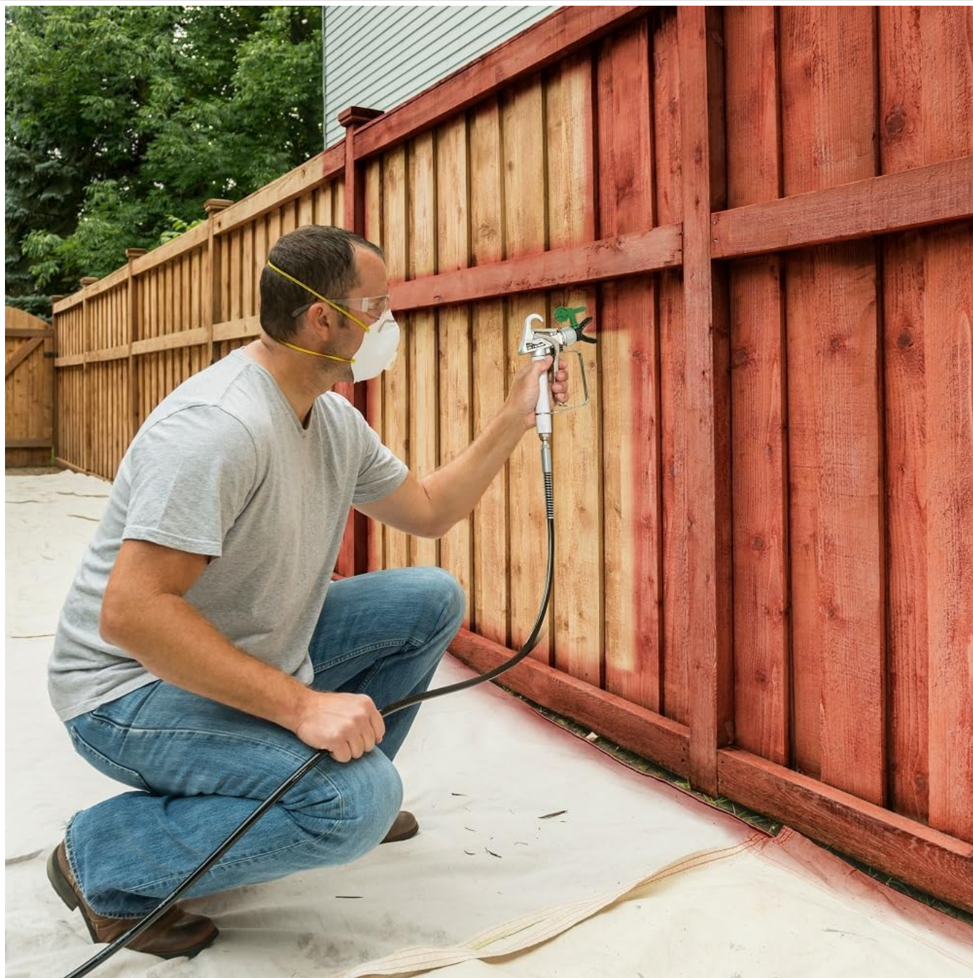
Image: A man staining a wooden fence, demonstrating the sprayer's utility for vertical surfaces and outdoor structures.
