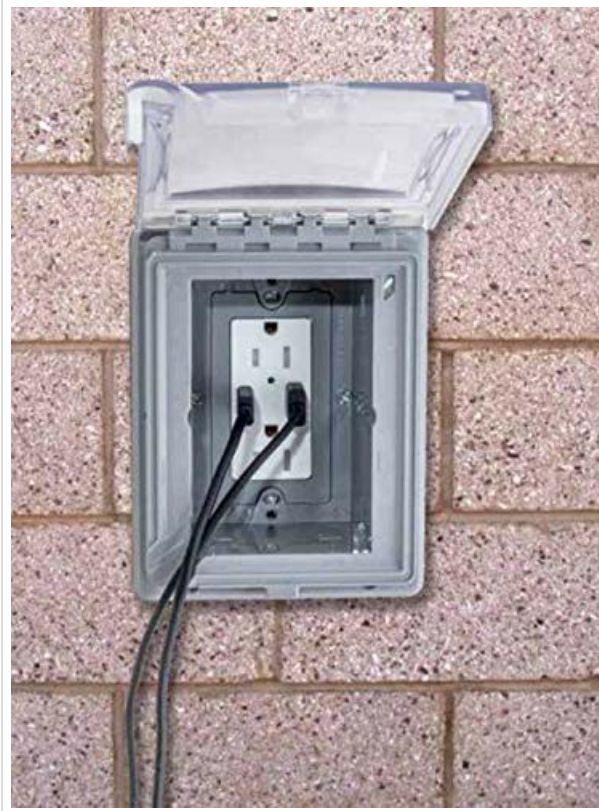
Image 2: This image illustrates the Hubbell Weather-Resistant USB Charging Outlet installed within a gray outdoor weather-resistant electrical box. The box has a clear cover, which is open, and two electrical cords are plugged into the AC receptacles of the outlet. This setup demonstrates how the outlet is protected for outdoor use.
