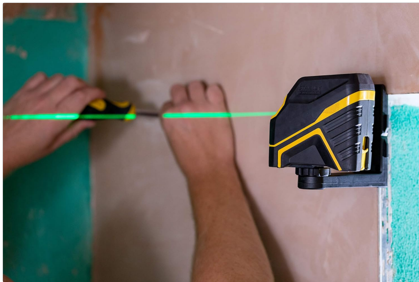
Figure 3: Laser level mounted using an L-bracket, projecting a horizontal line for alignment.
