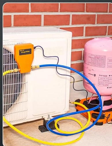
Refrigerant Recovery and Charging
