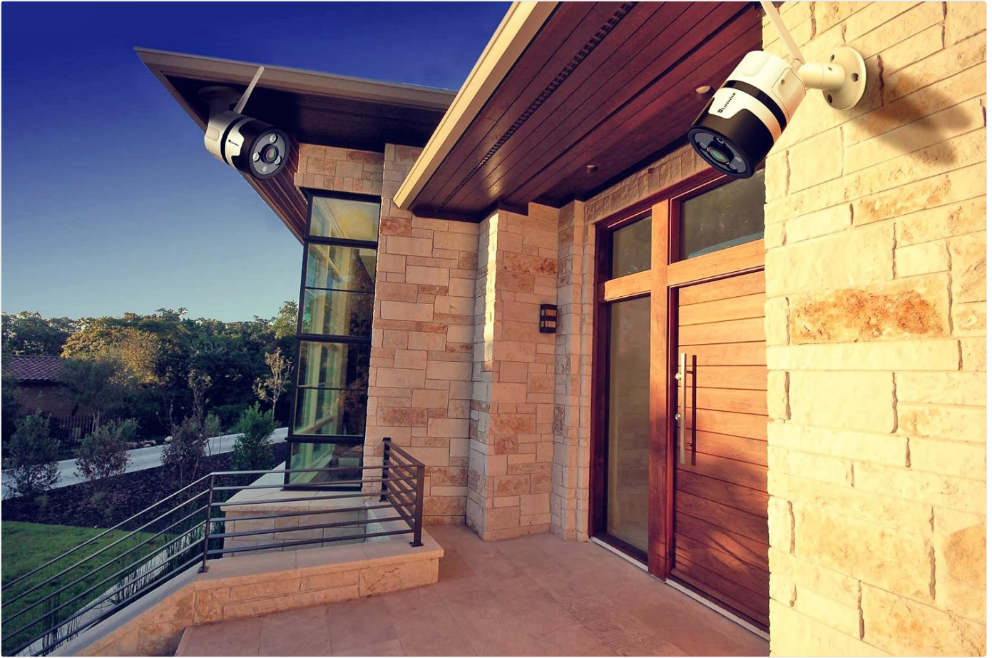
Figure 4.1: Example of outdoor camera installation on a building exterior.
