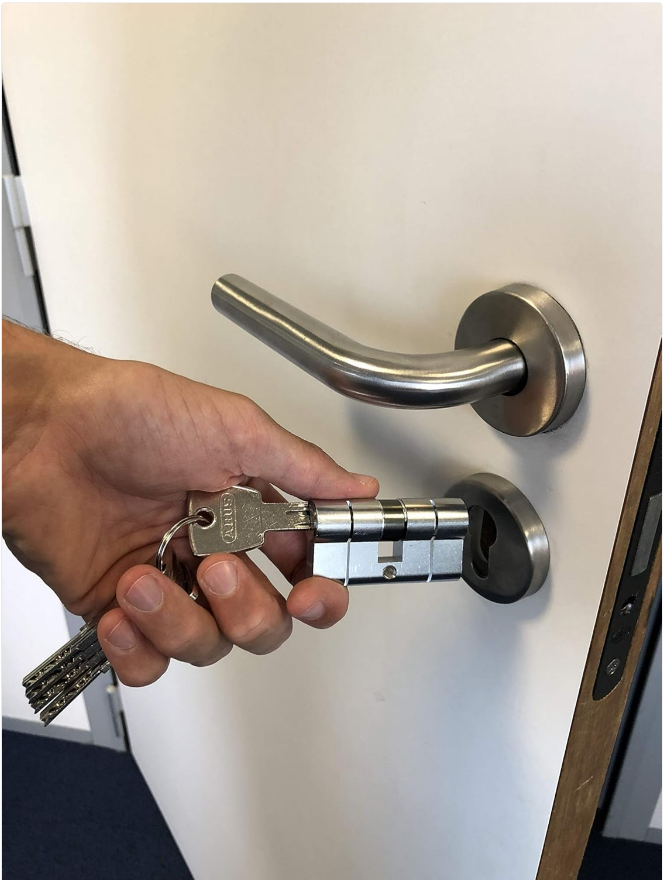
Image 5.1: Demonstrating the cylinder being aligned for insertion into a door lock.
