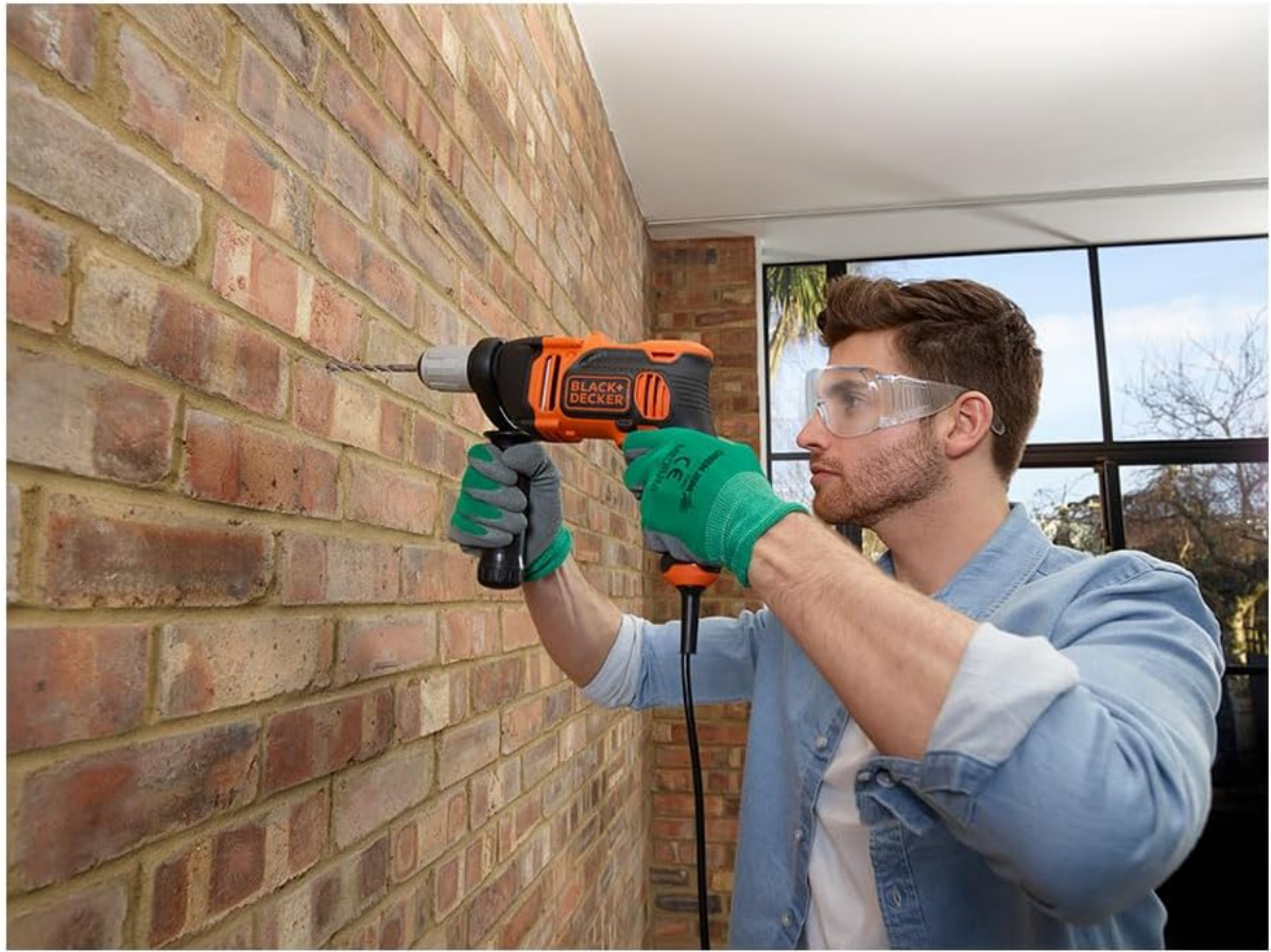
Figure 3: Demonstrating drilling into a brick wall using the hammer drill. Ensure a firm grip and proper safety gear.
