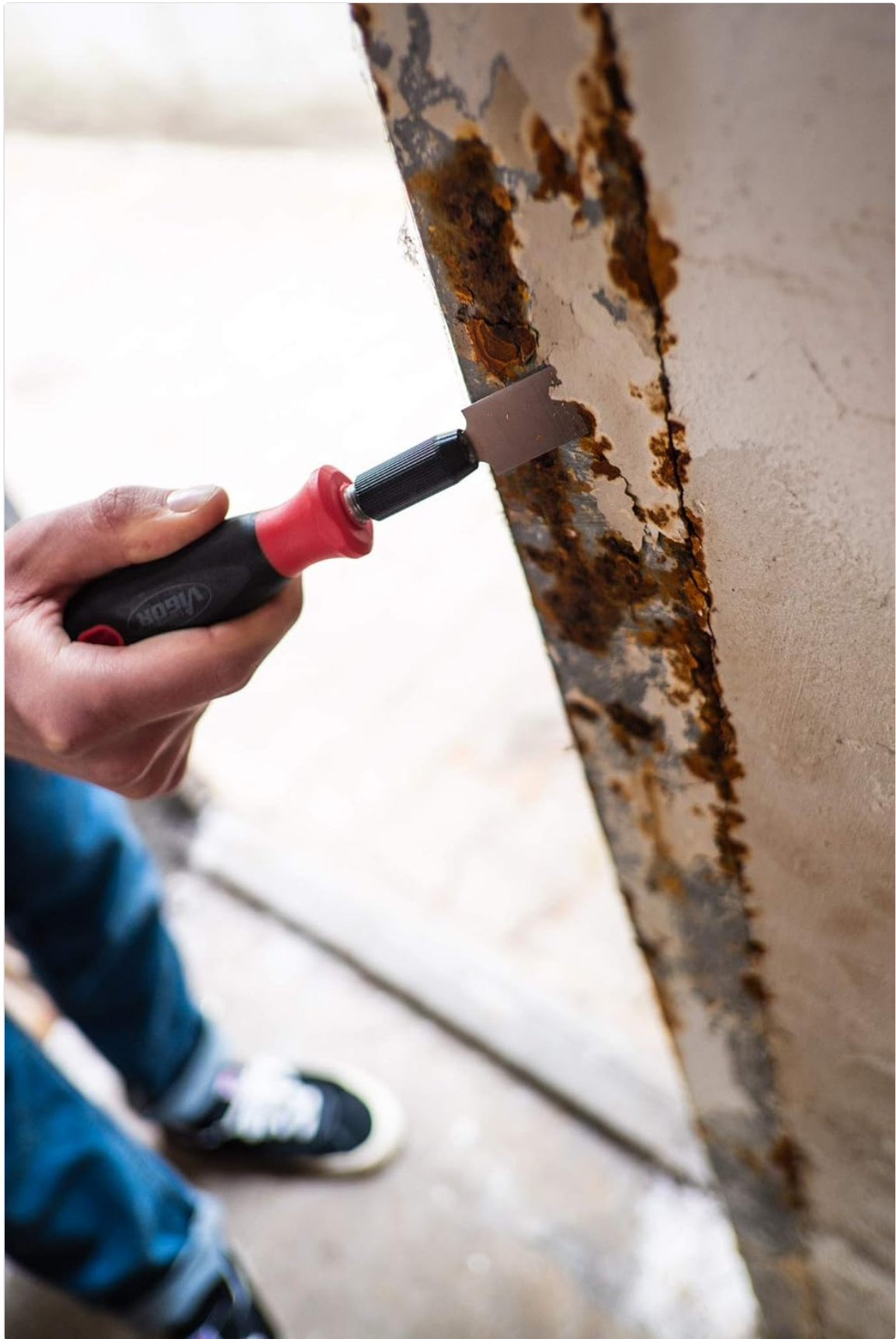
Image 4.4: Scraper being used to clean rust from a metal surface.
