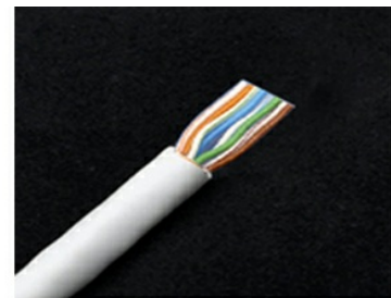
3. Separate wires and arrange based on T568A/B.
