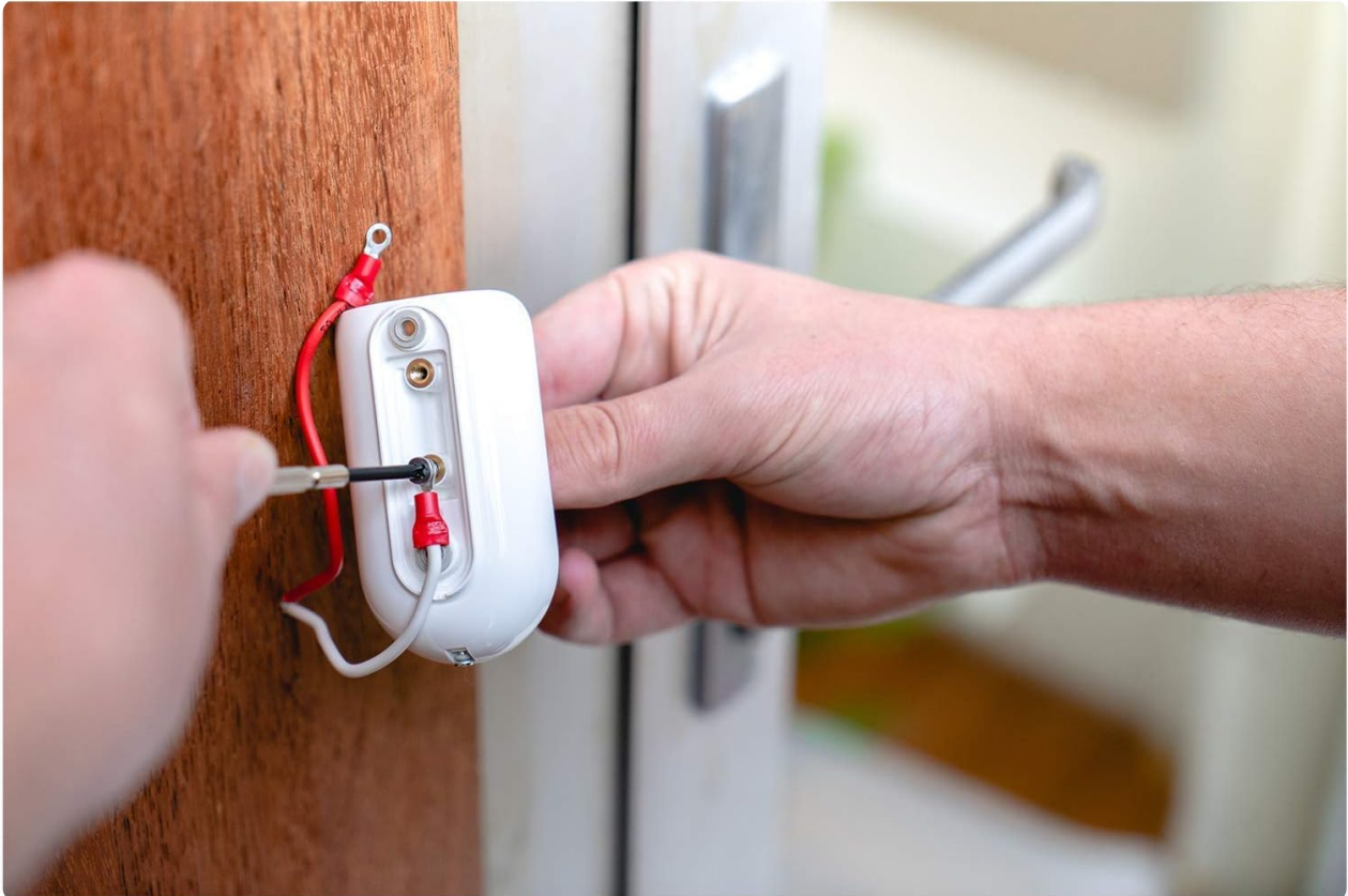
Figure 2: Installation of the doorbell's mounting plate using a screwdriver.
