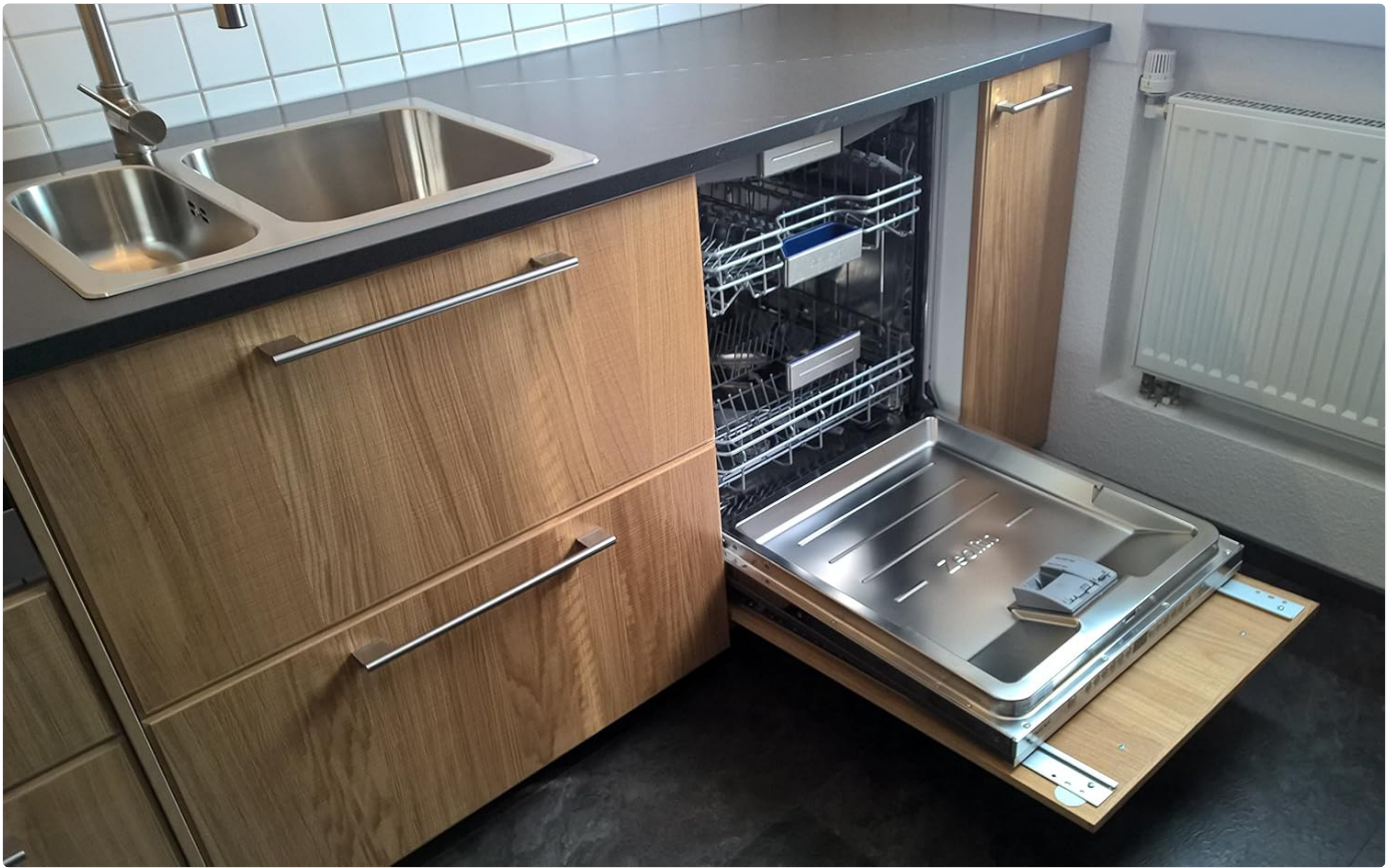
Figure 4.1: A fully integrated dishwasher installed in a kitchen cabinet, with the door open, revealing the interior and the sliding hinge mechanism at the bottom.
