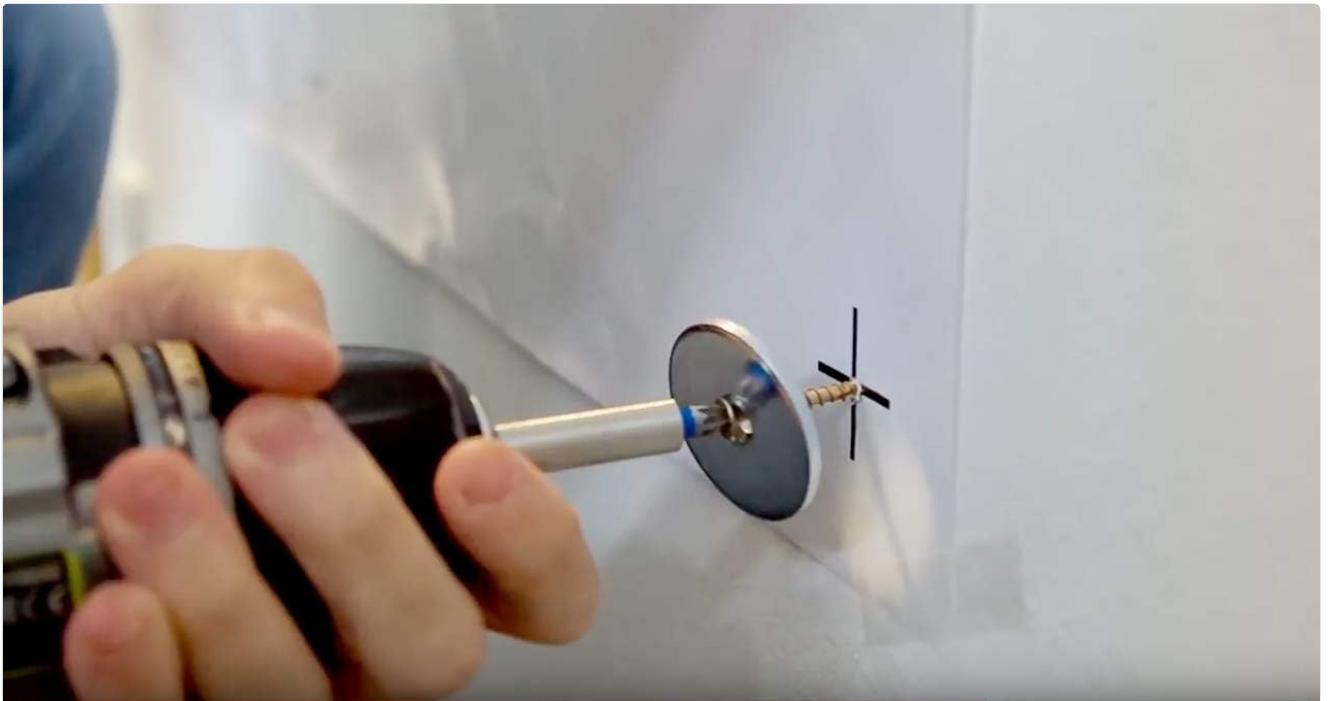
Image: Illustrates the process of drilling and securing the mounting hardware to the wall.
