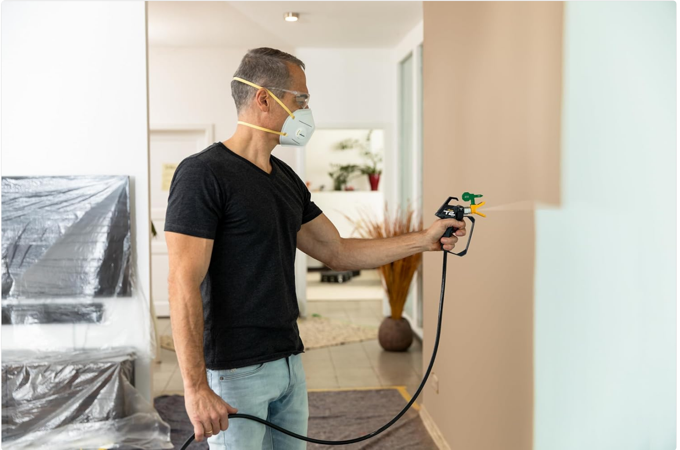
Figure 4: An individual applying paint to an interior wall, demonstrating the ease of use and mobility provided by the long hose of the Wagner Airless Control 150 M.
