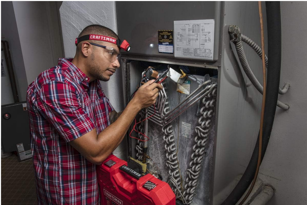
Image: Headlamp assisting with maintenance on an HVAC unit.
