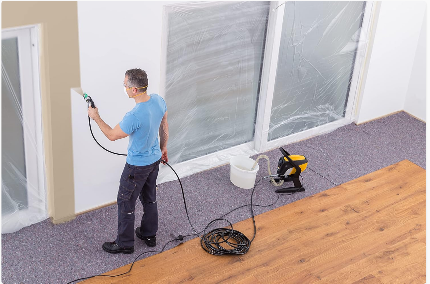
Image: A user setting up the spray system indoors, with furniture and floors protected by covers.
