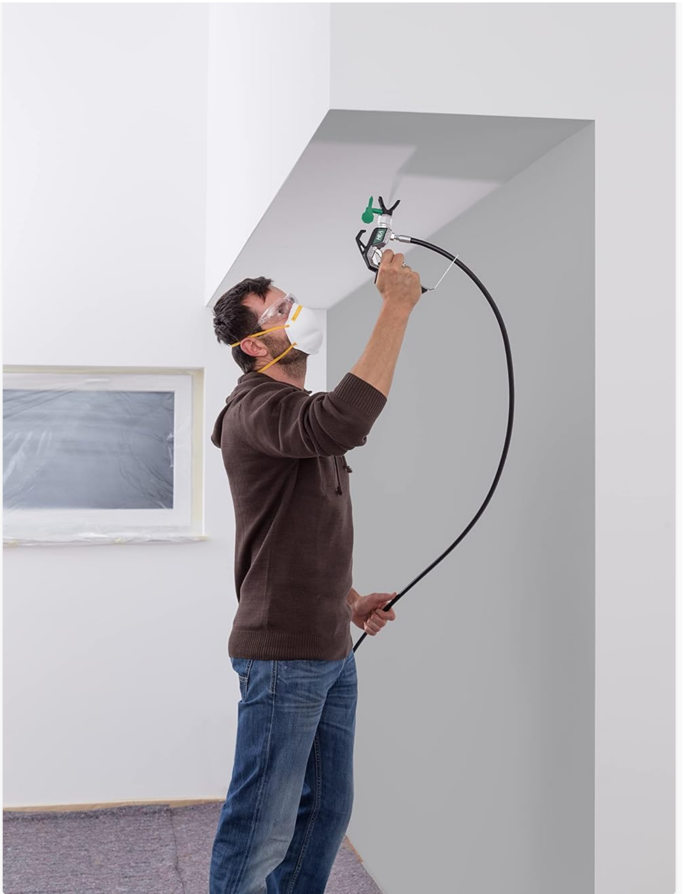
Image: A user applying paint to an interior wall using the Wagner spray system, demonstrating proper technique.
