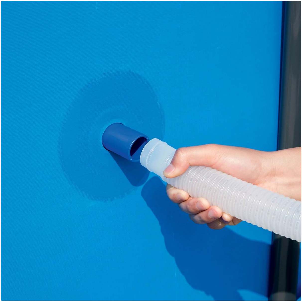
Image 4.1: Connecting a hose to the pool's return inlet.
