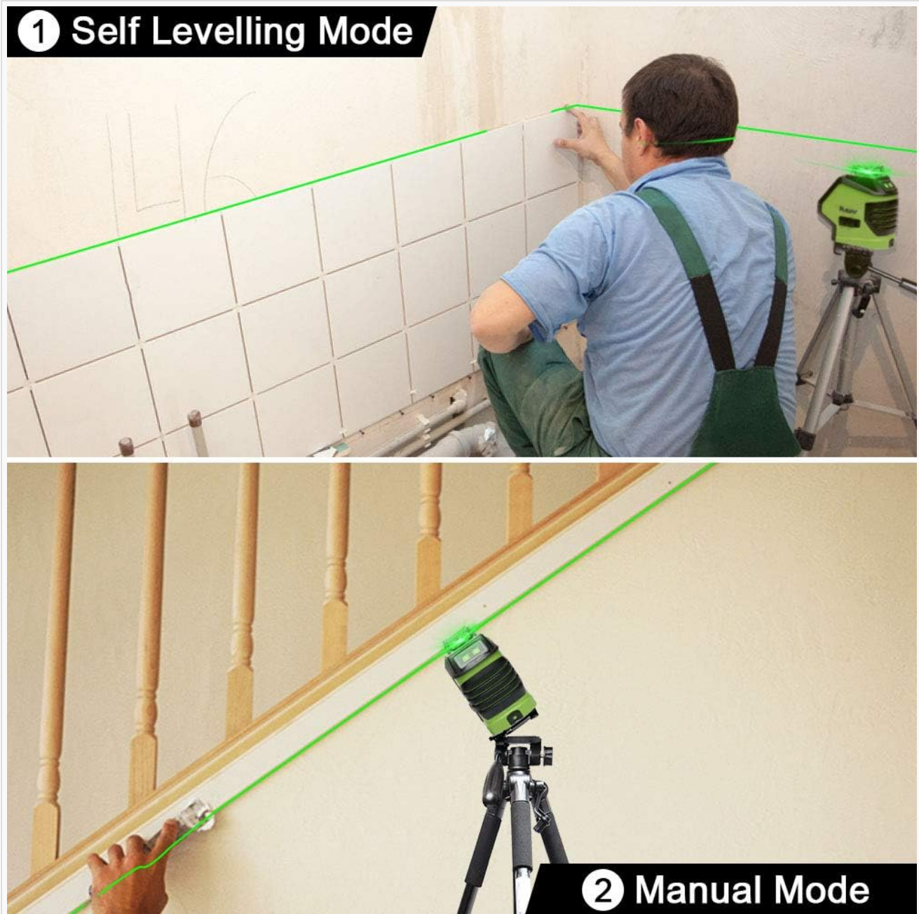
Figure 4.1: Using the laser level in self-leveling mode for tile installation.
